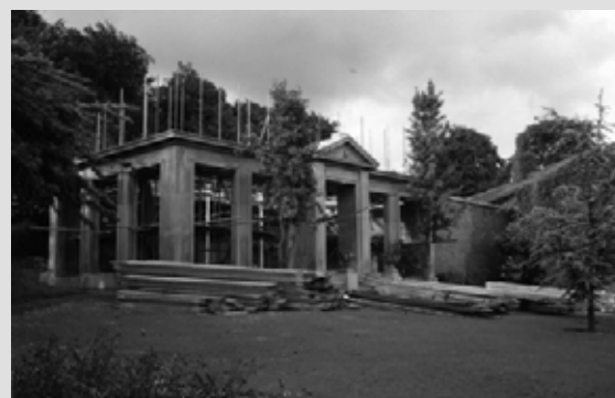
Photograph of the Conservatory, Philips Park, June, 1990 (IP). The architectural stone-work of the Grade II Listed conservatory was reconstructed at a cost of £140,000 in 1990. Unfortunately, the 'wrong kind' of roof was installed and inappropriate lighting introduced. There were calls for the retention of the cast iron columns and floor grilles as important features of the listed building. The conservatory has yet to be put to use!
