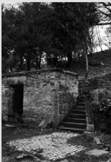
Photograph of forcing tunnel, Philips Park, April, 1995 (IP). This row of three brick-faced chambers (shown on the pre-1833 plan) was exposed during ground work for the Philips Park Management Plan of 1995.
