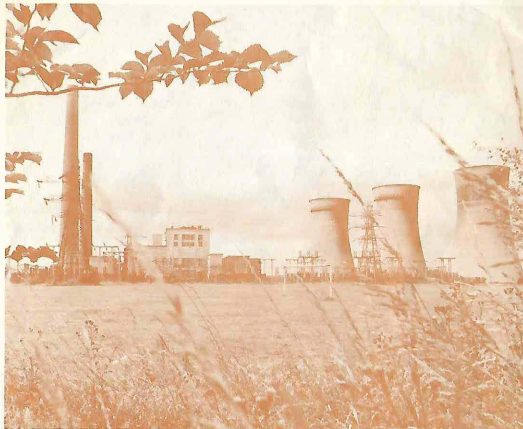
Agecroft Power Station
